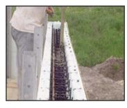
method is also subject to thermal bridging where outside cold seeps in to cause uncomfortable cold spots, drafts, and mustiness. On the other hand, the Nudura concrete walls have shown to deliver energy savings of up to 70 percent and delivers a building envelope up to three times more sound resistant, four times more fire resistant, and nine times stronger. Floor and ceiling construction is now advanced too. More information is available online at www.nudura.com.
